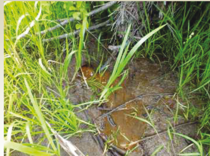
Figure 4- 36 : Drain non protégé
