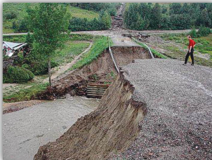
Photo 5 : Remblai routier effondré, 6 e Rang, Tingwick
