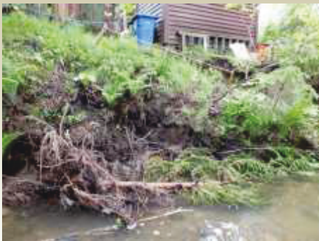
C. Berge effondrée
