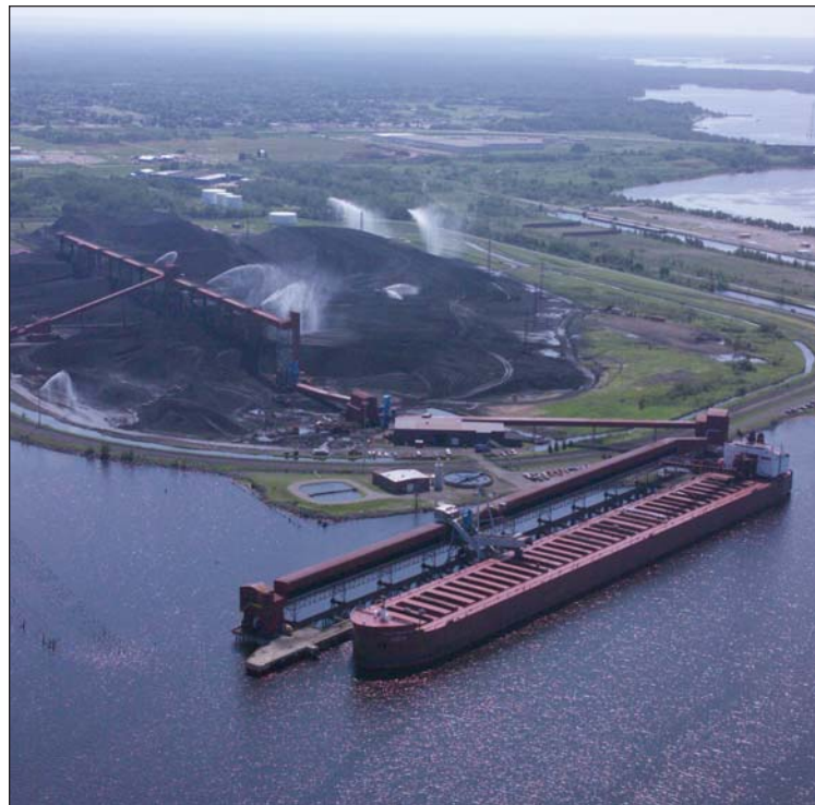
Terminal Midwest Energy, Superior (Wisconsin) Source : http://www.midwestenergy.com
